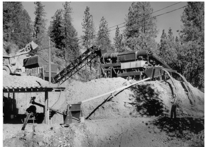
Photo 19. View of TRI-R Engineering's recovery system at the Stinson Mine. Ore is loaded by backhoe into the feed bin, then delivered by conveyor to the trammel. The discharge is coming from the light colored primary concentrators. Concentrates are stored in the sump at left, then processed in the helix.
