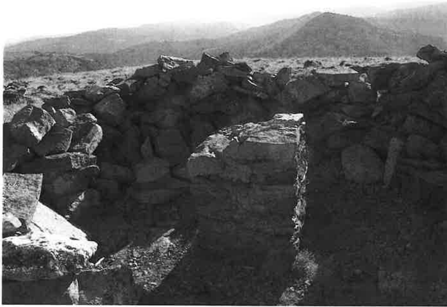
Mt. Lola Summit Foundations of Heliotrope Pedestal
