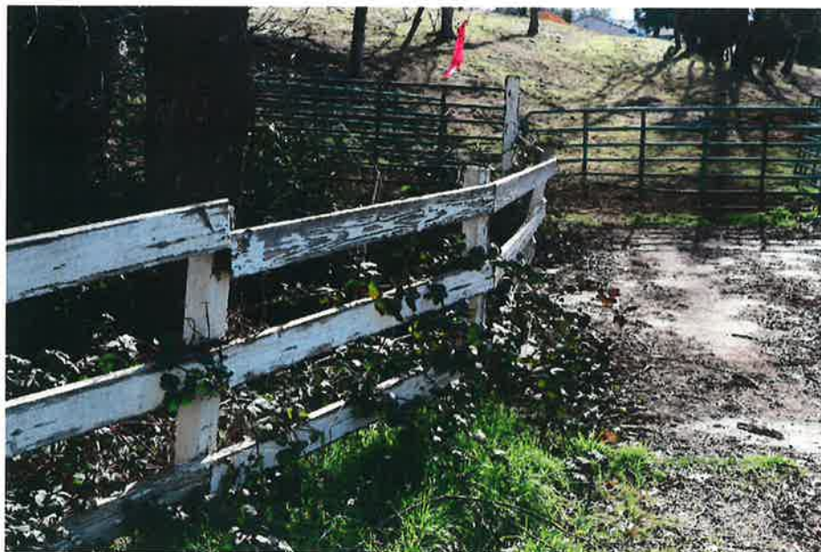
4B. View to the east showing the existing road and bridge over French Ravine Creek. The new, encased pipe will be adjacent to the existing bridge, and the new leach field will be on the sloping hillside behind the green gate shown in this photograph.
