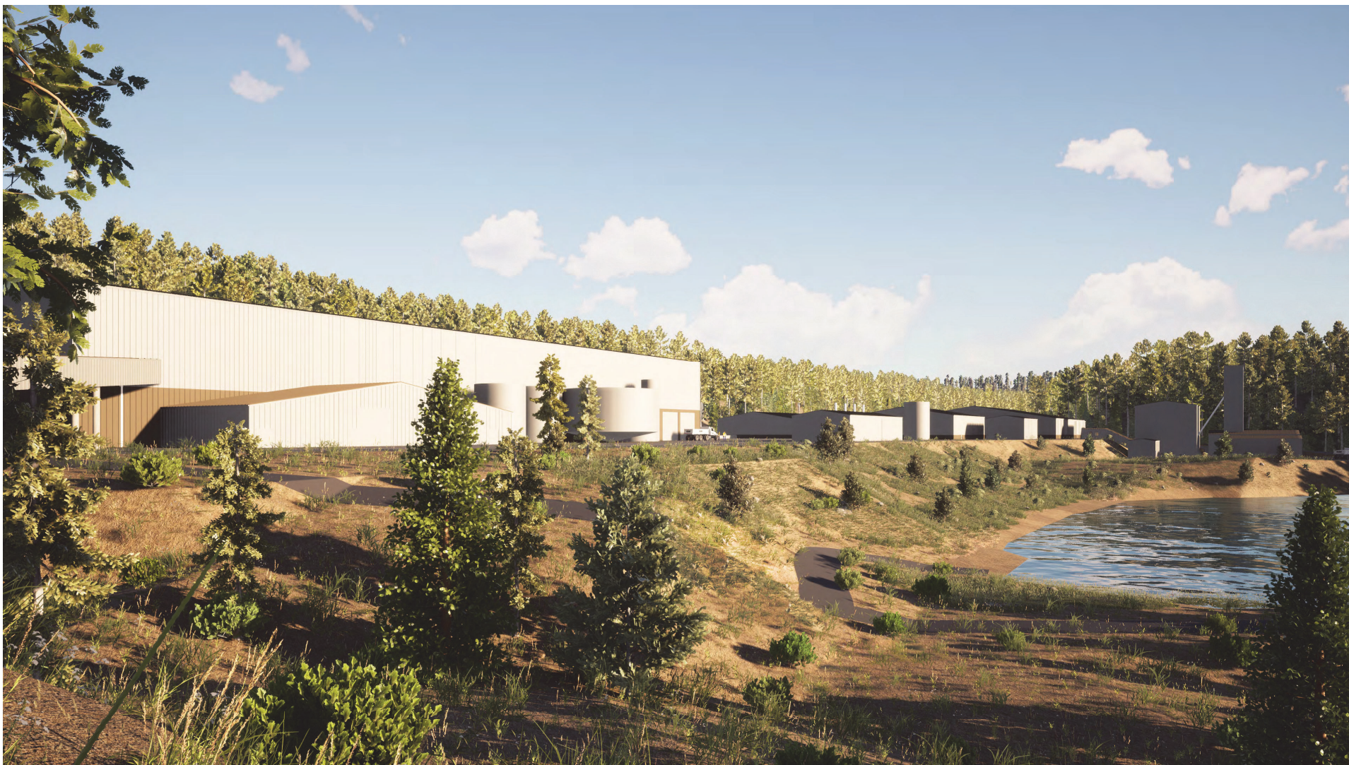
④ PROCESSING PLANT (WEST)
