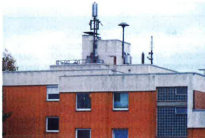
Fig. 1: Cell Phone Transmitters on Top of the Multistory Building at Feldstraße 28, Selbitz, Upper Franconia
