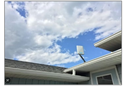
Figure 2-1 Roof-Mounted Fixed-Wireless Equipment
