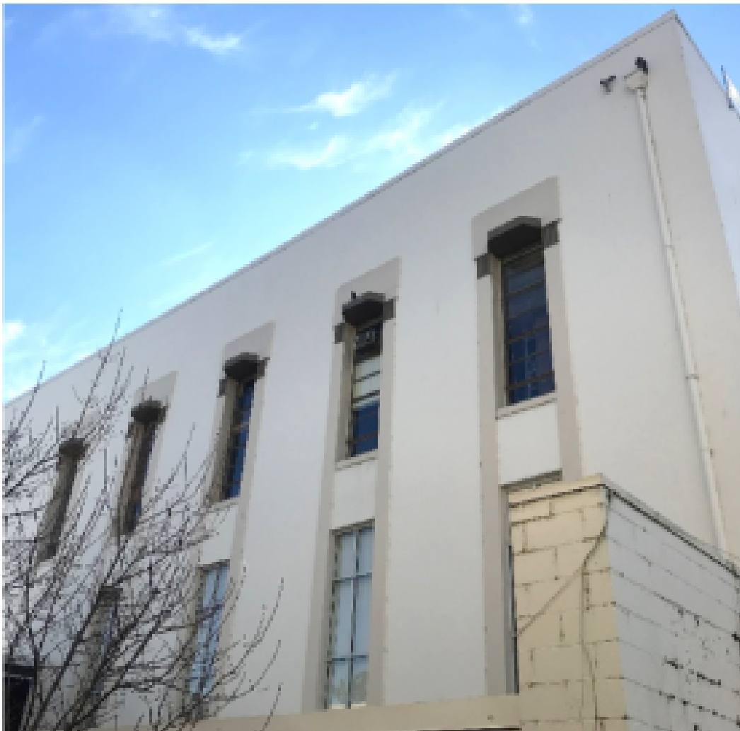
Figure 9. East facade, view southwest fenestration pattern and material, including replacement second-floor windows and CMU enclosure (ARG, 2022)
