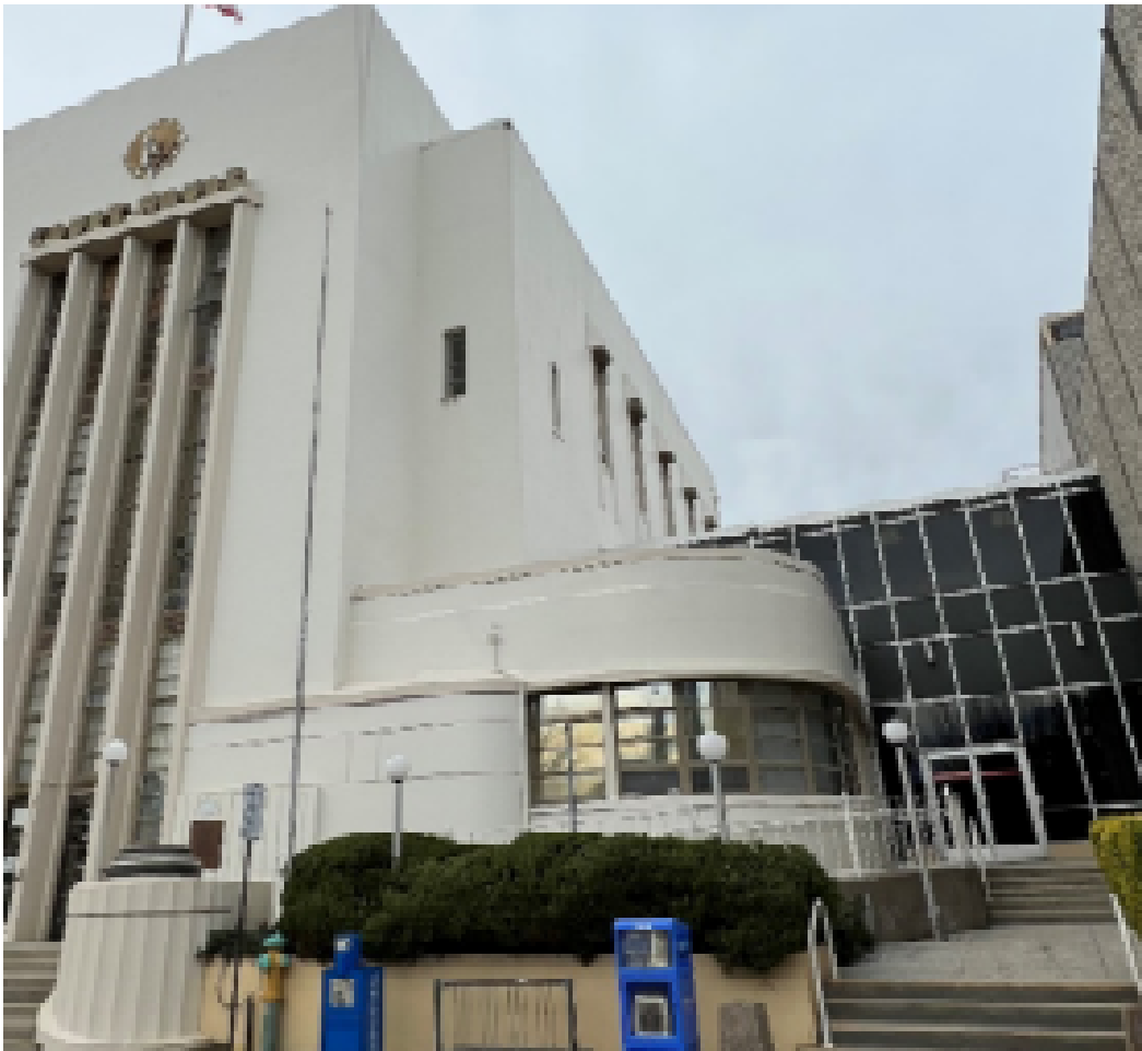
Figure 11. Primary (south) and east facades, view northwest, showing 1937-constructed elements including first-floor volumes and entry details, and 1964-constructed connecting corridor to the Annex (at right) (ARG, 2022)
