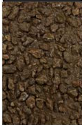
Equipment Cabinet Roof Material
