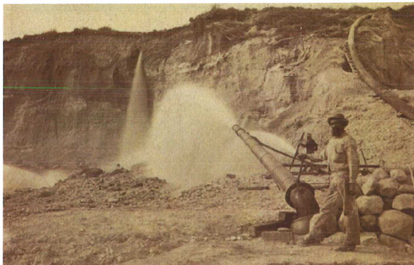
Hydraulic Mining at Malakoff Diggins, 1874
