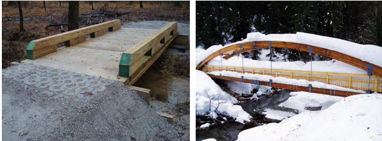
Figure 7: Example of a minor trail bridge design (left) and a major trail bridge design (right) both designed to be aesthetically pleasing and to withstand heavy snow loads.(photo credit USDA Forest Service, National Technology and Development Program).
