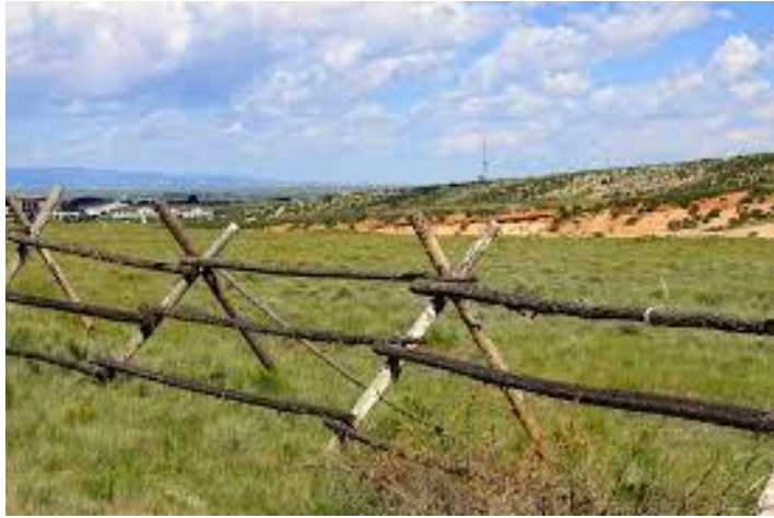
Figure 9: Example of buck and rail- style fencing that is built to withstand snow loads.
