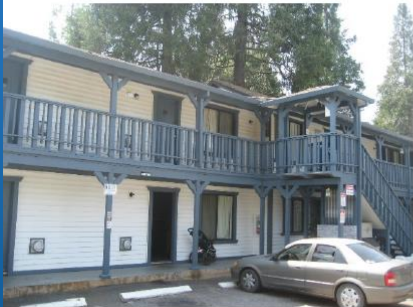
Southern wing of the motel
