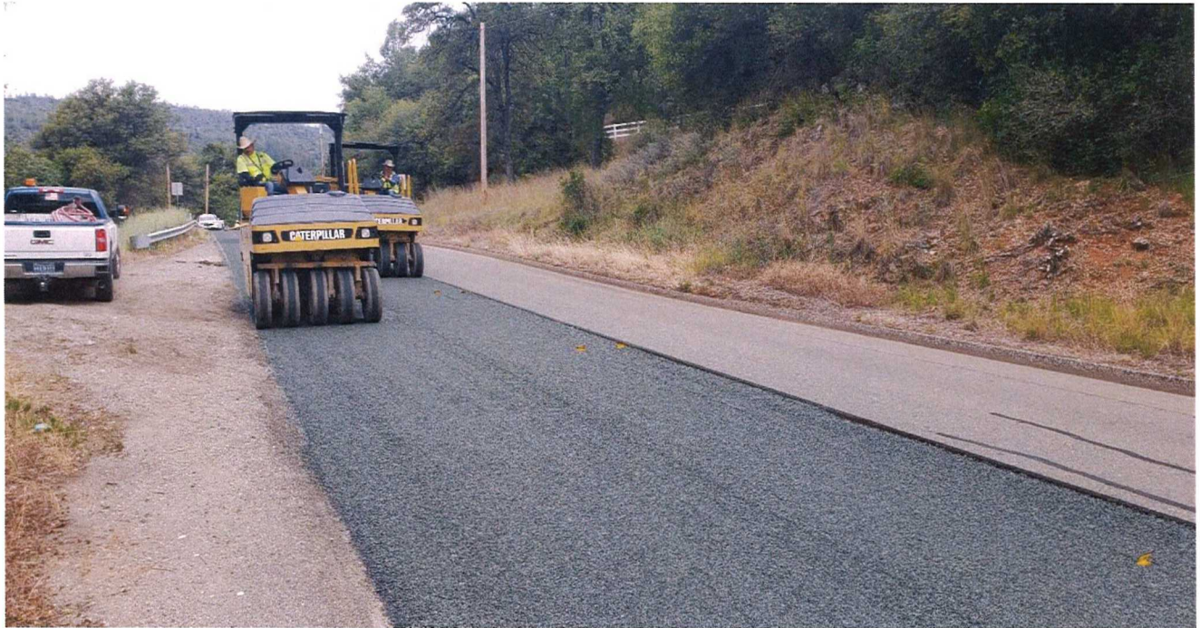
Placing chip seal in Alta Sierra
