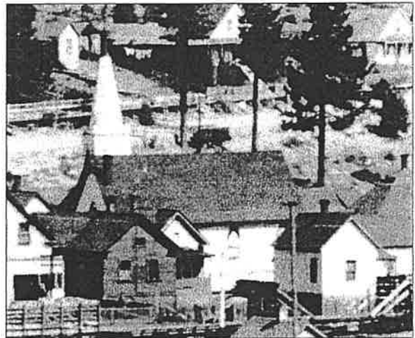
A turn-of-the-century image of the United Methodist Church and early residences demonstrates the pervasive use of wood lap siding.
