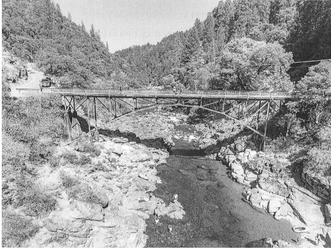
Edwards Crossing Bridge
