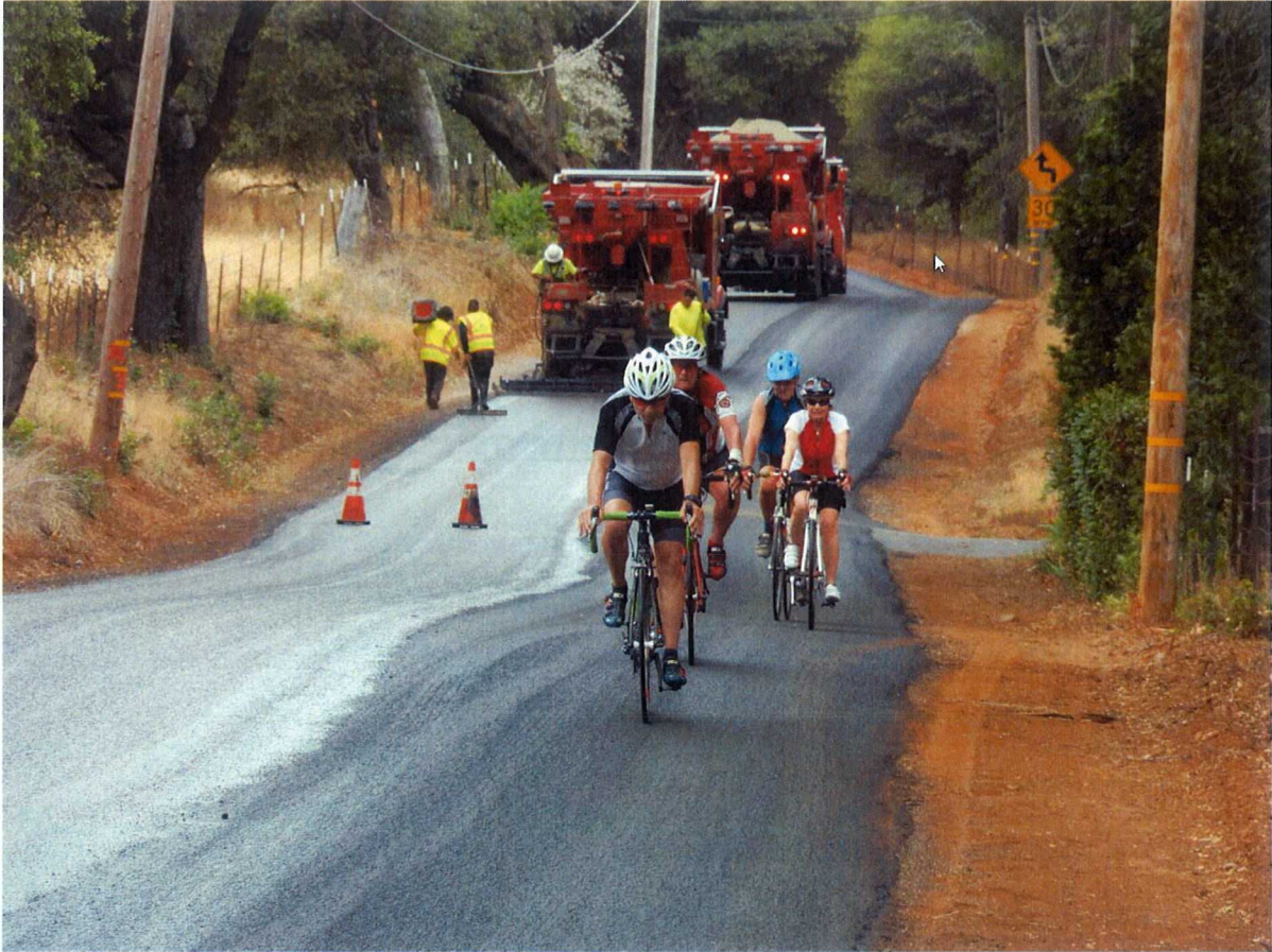
Bicyclists Traveling Through the 2018 Road Rehabilitation Project
