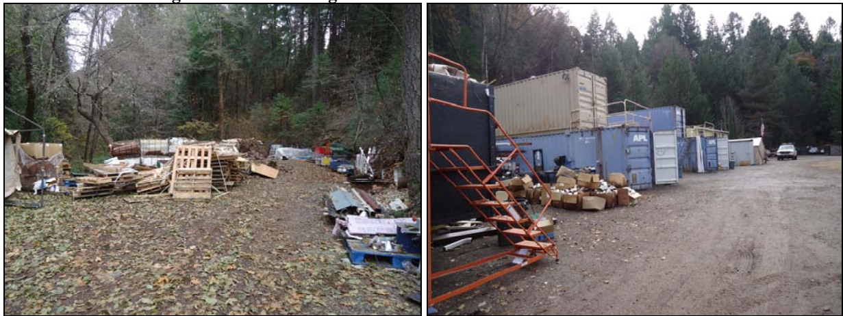
Figures 4 and 5. Storage containers and loose materials stored onsite
