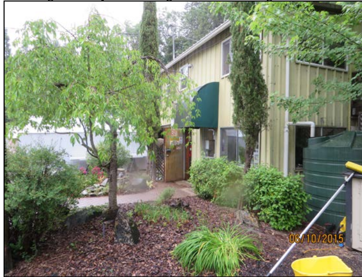
Figure 6: Byers existing office and storage structure
