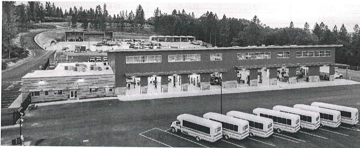
Figure 2 Nevada County Operations Center
