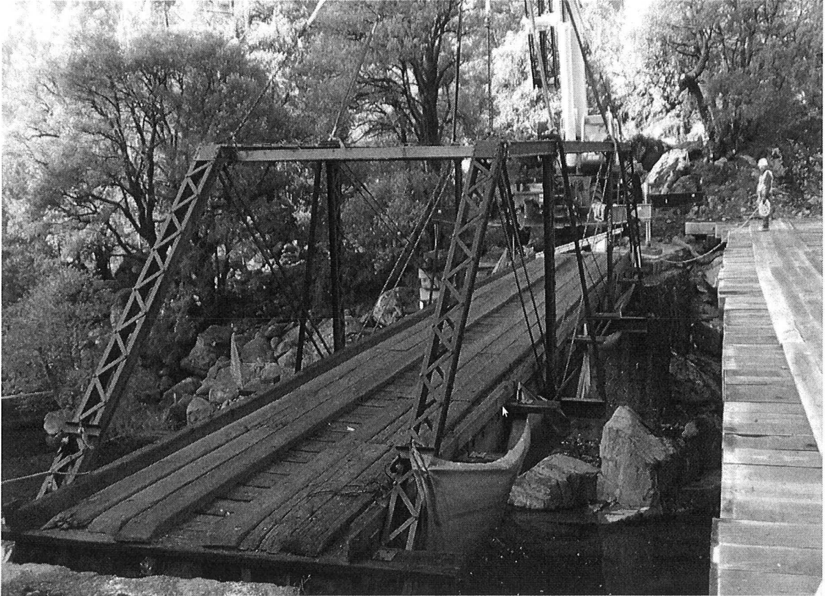
2016 MAYBERT ROAD BRIDGE REPLACEMENT PROJECT
