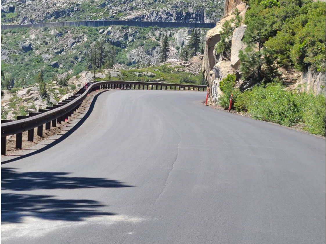
Widening Donner Pass Road
