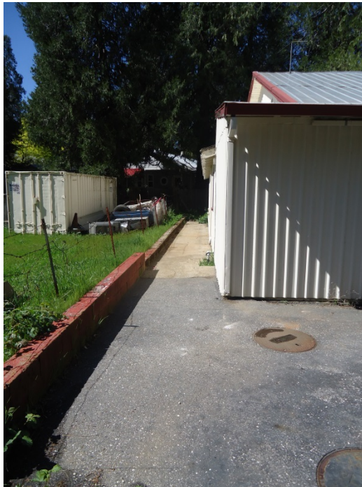
Western View of Rear Prop. Line
