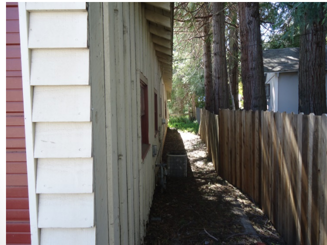
Southern View down Western Prop. Line
