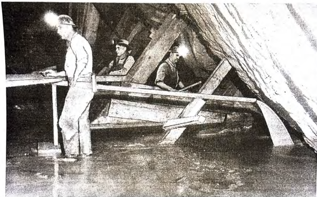
FRESH SAND-SLIME FILL is solid enough to permit the operator Raymond Coulter to stand on it. The fill is discharging from the pipeline at the right. In the background, two miners are just completing a cribbed raise that comes up through the fill.
