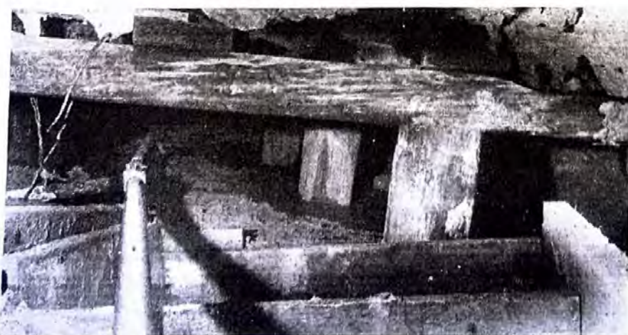
TAILINGS FILL close to back of old timbered stope. In foreground is timbered raise. Stretching away from camera is pipeline that conveys the sand-slime fill.
