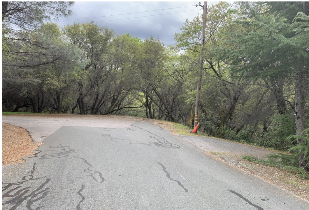
Figure 5: Looking South at Northerly Boundary on Rodeo Flat Road
