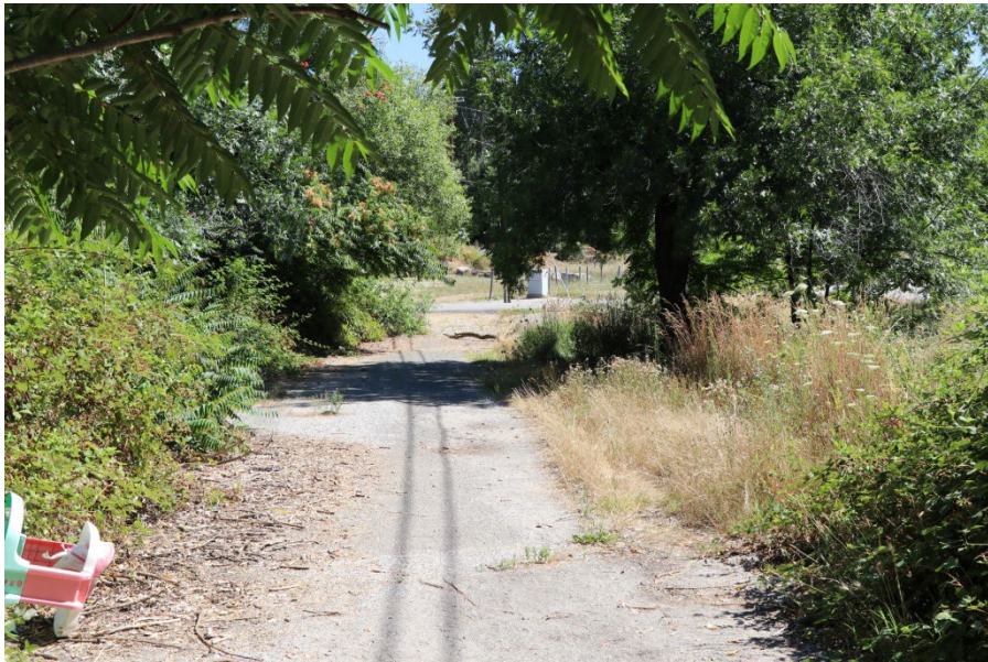
4F. View of the abandoned road near the Community Center where the new pipeline will be installed adjacent to the riparian vegetation.
