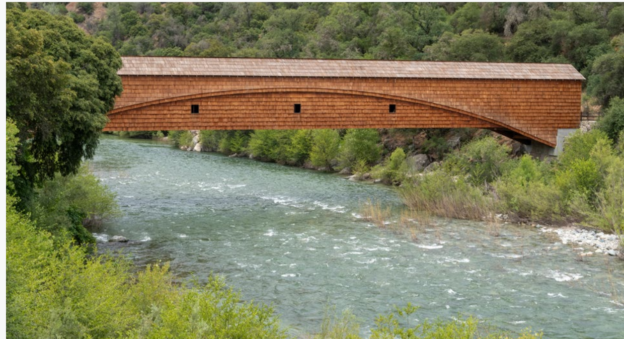
Bridgeport bridge over the South Yuba River
