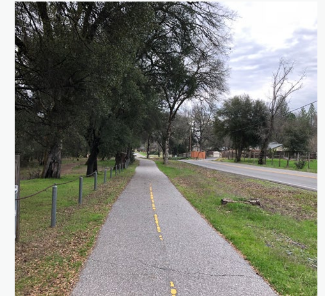
Shared-use path adjacent Western Gateway Regional Park
