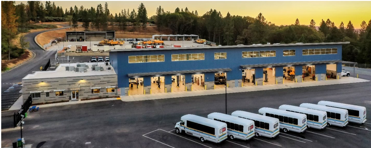
Figure 2 Nevada County Operations Center
