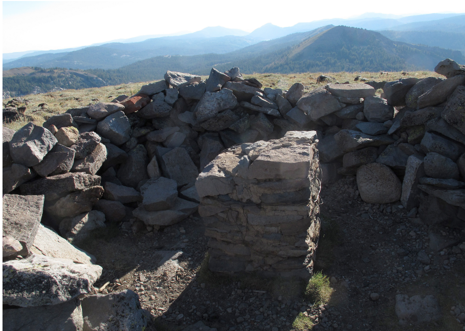
Mt. Lola Summit Foundations of Heliotrope Pedestal
