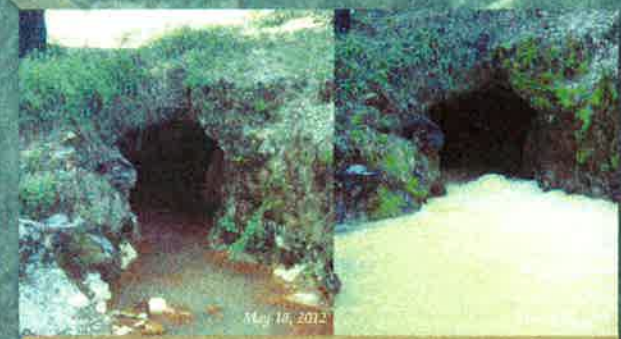
Hiller Tunnel Discharge at Low and High Flow: Hiller Tunnel is the only visible surface water discharge location of the Malakoff Diggins pit. It has year round flow, and discharges vast amounts of turbid water during storm events.
