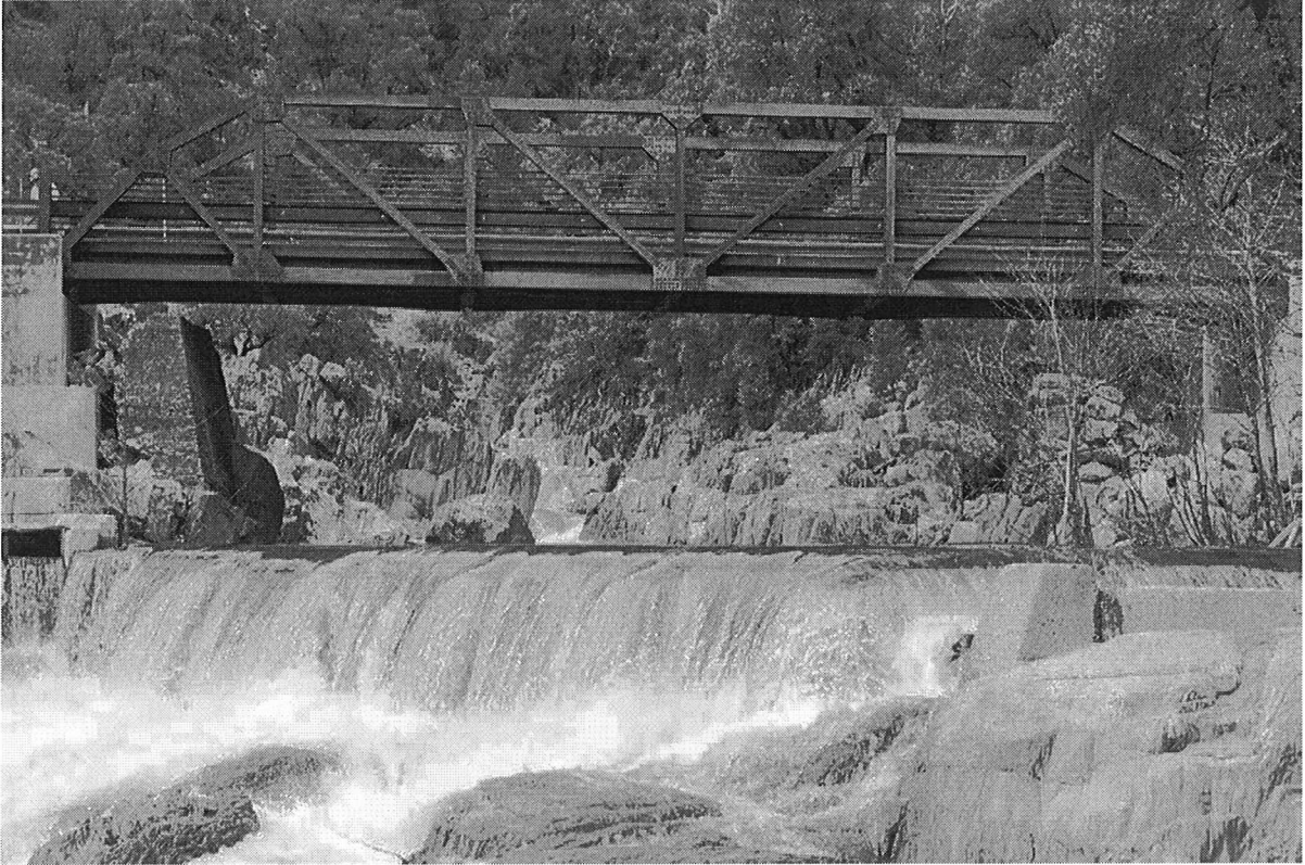
COMPLETION OF THE 2016-17 MAYBERT ROAD BRIDGE PROJECT
