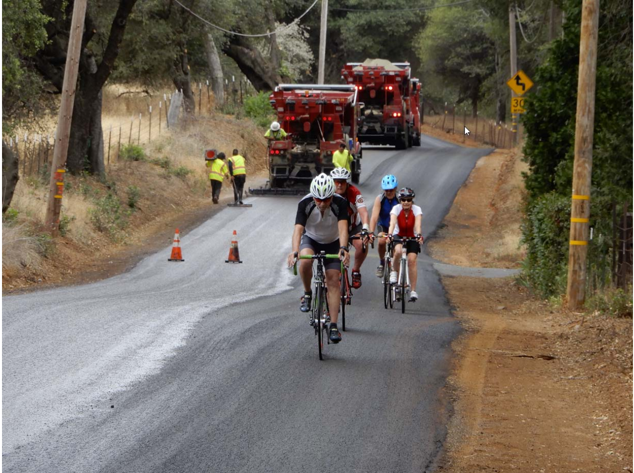
Bicyclists Traveling Through the 2018 Road Rehabilitation Project
