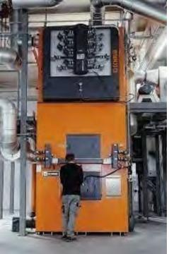
Figure 19: Proposed Wood Chip Boiler
