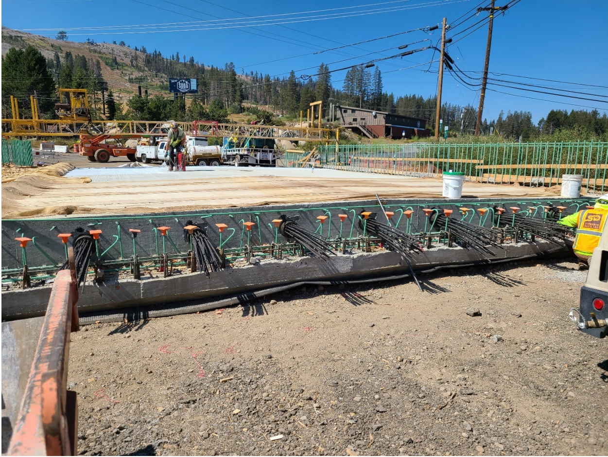
Placing rebar in the Soda Springs Road bridge
