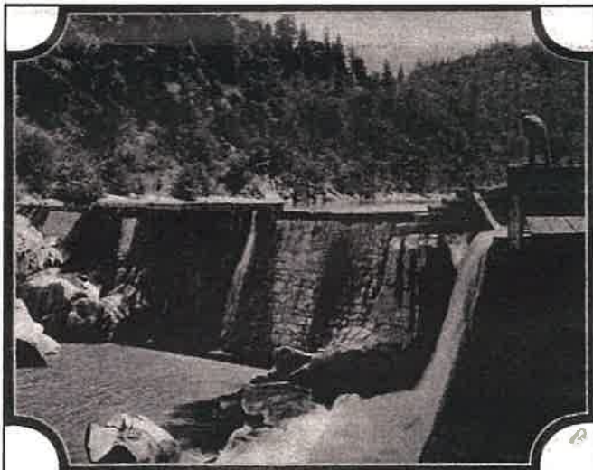
The diversion Dam for the first powerhouse was located 3&1/2 miles above the powerhouse on the South Yuba River.
