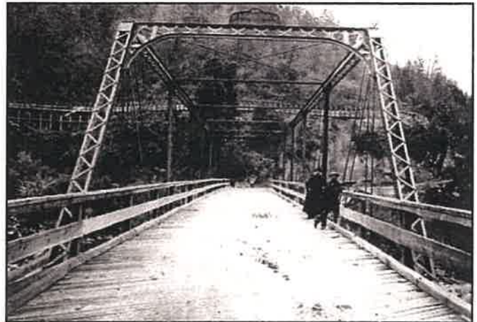
This view from the north side of the Purdon Crossing Bridge, shows the Nevada Flume on the slope above it on the south side.
