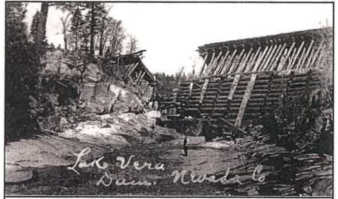
The Lake Vera Dam was originally 54 feet high and it failed in early 1905, as this photo shows.
