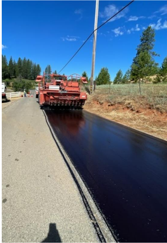
Before, during, and after of micro surfacing on Empress Rd
