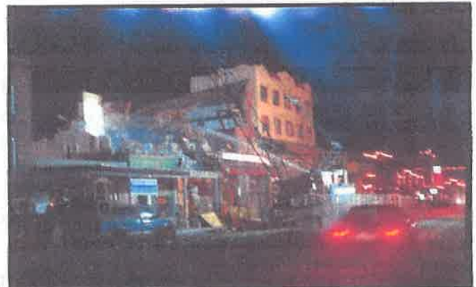
(Above) Masonic Lodge after 1993 Propane Explosion; COR2344
