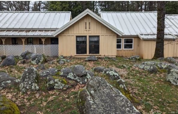
San Juan Ridge school building
