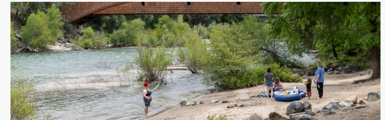
▼ Bridgeport covered bridge and river access
