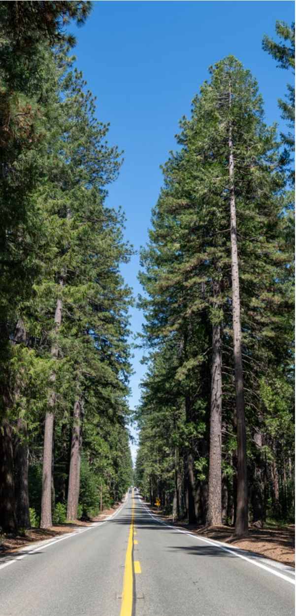
Highway 20 in Nevada County
