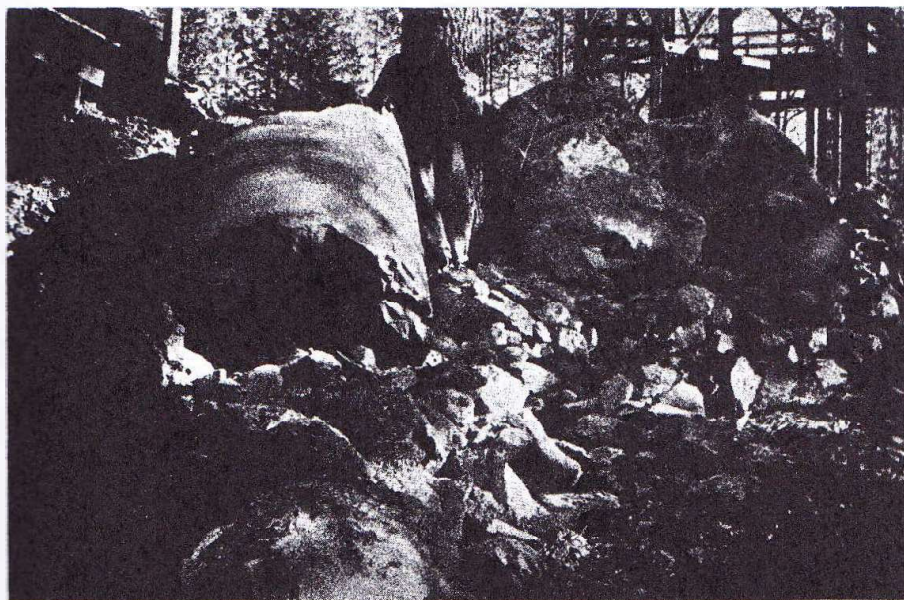
Core sections (5 ft. diameter) from Newsome shaft-boring machine at Brunswick Mine of Idaho-Maryland Group. Photo by Walter W. Bradley
