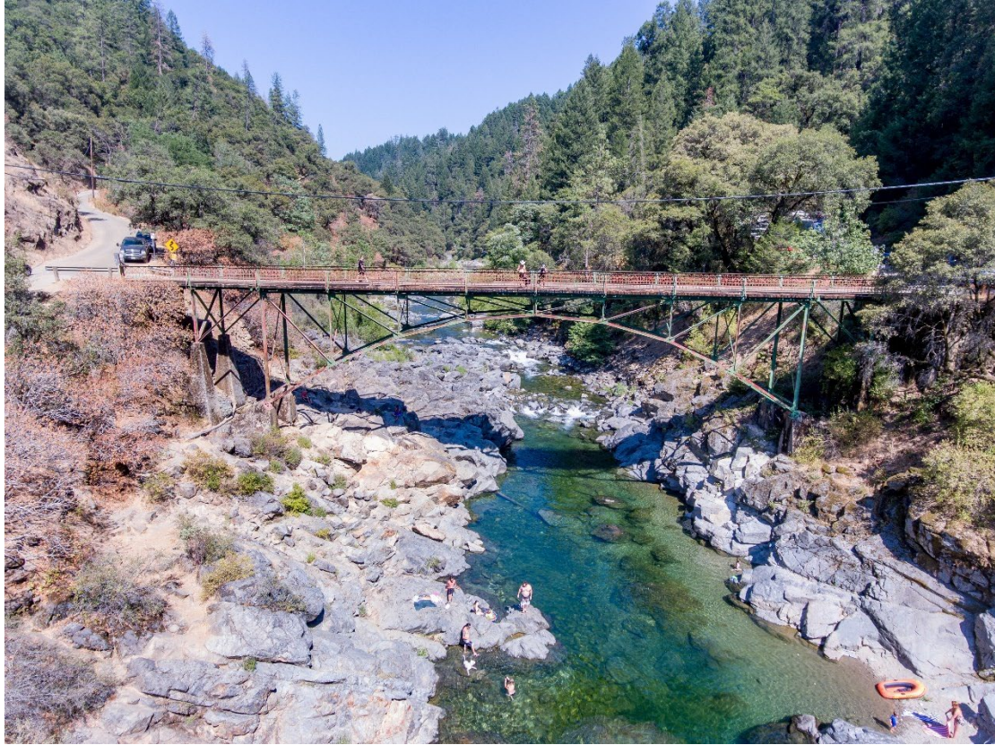
Edwards Crossing Bridge
