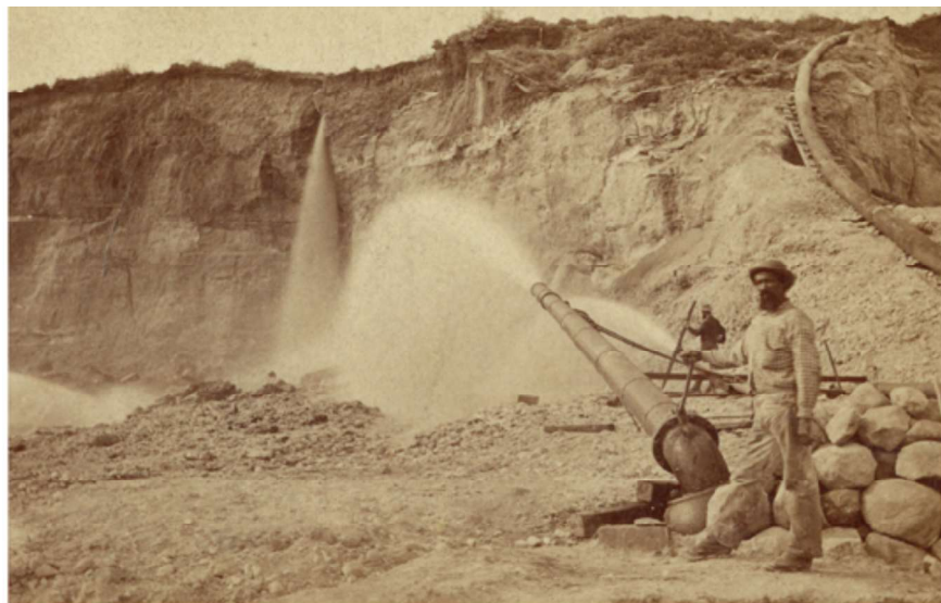
Hydraulic Mining at Malakoff Diggins, 1874
