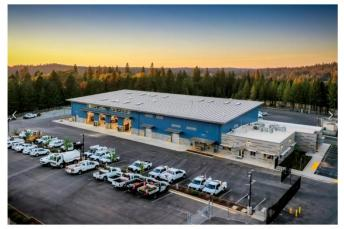
The completed NCOC includes a 5-acre laydown yard; parking for heavy equipment and transit fleet, vehicle wash building; sand barn; administration building, crew rooms and fleet maintenance operations; a flatbed pullthrough bay; 12 maintenance bays; 6,000-SF equipment platform; and roof structure for future photovoltaic array. CLIENT County of Nevada
