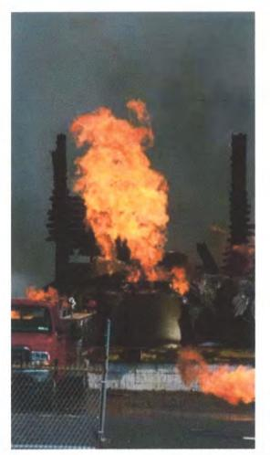
(4) These 250-pound cylinders vented to the atmosphere as efforts were diverted to save the town by cooling the fixed tanks.
