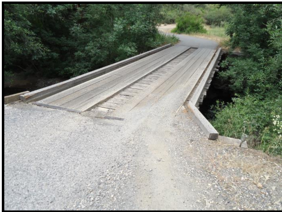
Figure 3: Private Bridge on Mulberry Lane
