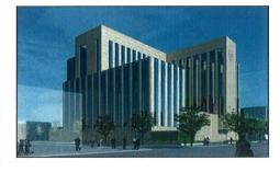
Type I-A fully sprinkled construction, with an estimated total cost of \$233 million. The total area of the courthouse building is 233,695 square feet. The courthouse building consists of a structural steel frame with exterior curtain wall. The courthouse building contains court rooms, jury chambers, judicial chambers, administrative office spaces, sallyports for security and other associated facilities.
