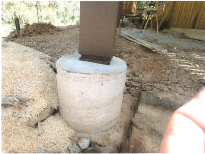
Every post is set on a metal stand-off base.
