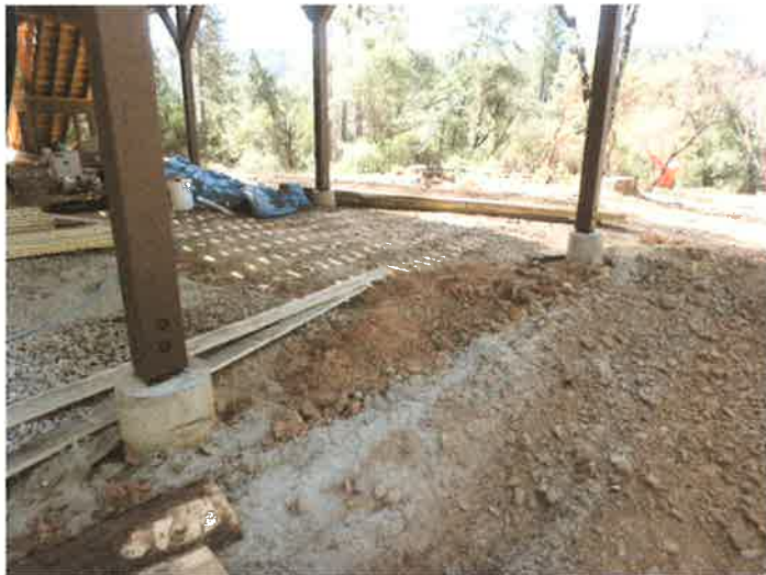
A concrete slab will extend past the piers.
