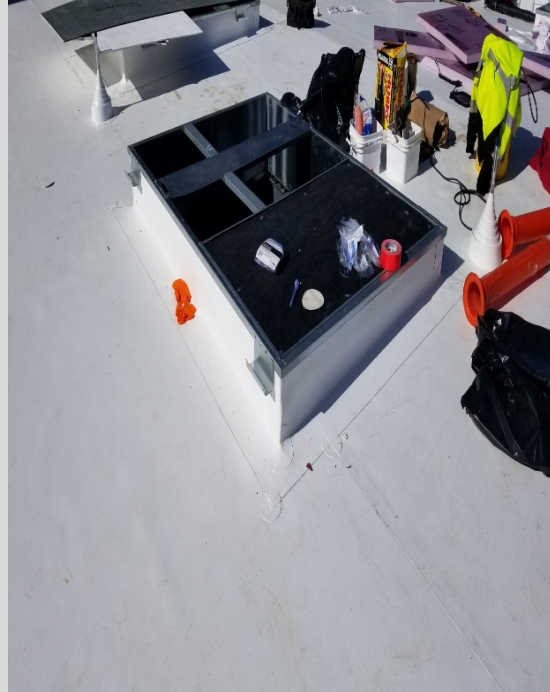
Photo 2 - Office Area TPO Roof Installation
