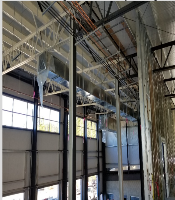
Photo 7 - Garage HVAC and Pipe Bridges
