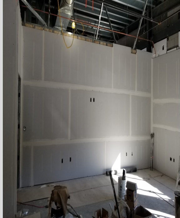
Photo 5 - Office Area Drywall Installation
