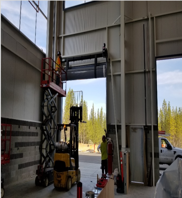
Photo 6 - Motorized O/H Door Installation
